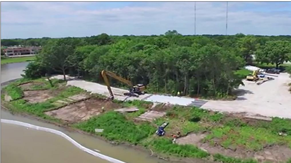
Contamination is removed using a carefully mapped grid pattern on the Milwaukee River above Estabrook Park Dam. Photo credit: Duane Thomas, EA Engineering.
