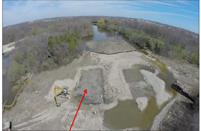
Temporary cofferdams allowed for dry excavation of the sediment. Photo shows main channel of Milwaukee River looking upstream (North). Photo credit: Duane Thomas, EA Engineering.
